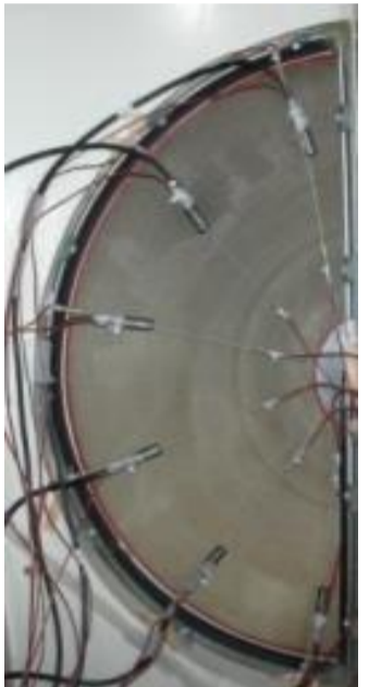
Appearance of desiccant air-conditioning system Desiccant wheel
