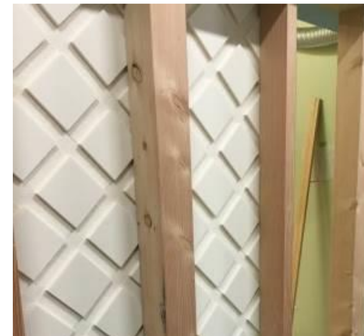
Figure 11 Aeration layer of air cycle board
