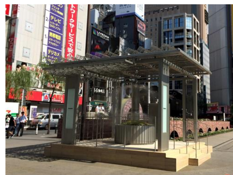
Mist spray system in Shimbashi, Tokyo
